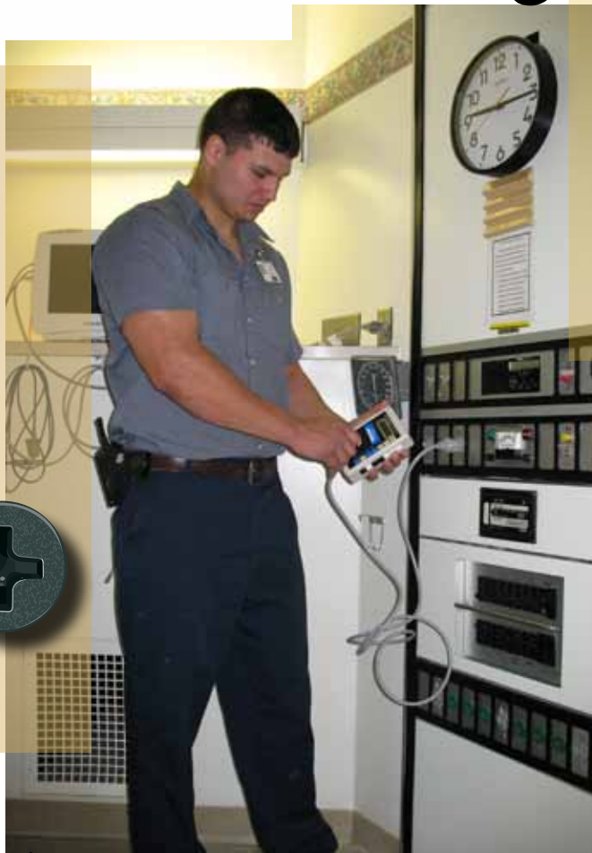
Darren Campos conducts a Line Isolation Monitor Test.
