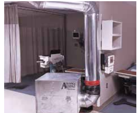
Maintenance staff installed a special HEPA filtered air scrubber to exhaust room air to the outside and create additional negative pressure space.
