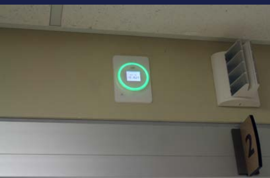
Each negative pressure room has a digital sensor that lights up when negative pressure has been achieved.
